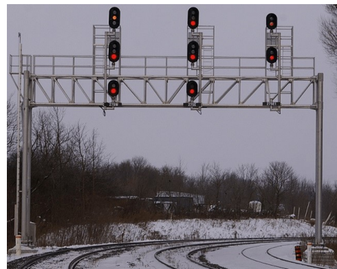
A bridge over three tracks at a CTC interlocking.
